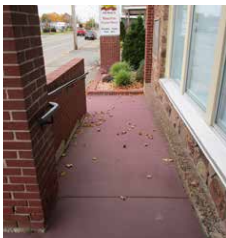
KA 19 | Ramp leading away from entrance
