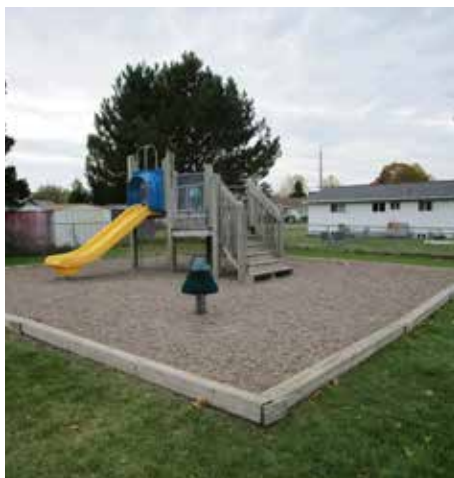
KA 13 | Typical unaccessible playground found throughout county
