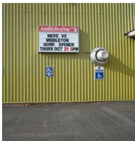
PA 5 | Accessible parking signage at Glooscap Arena
