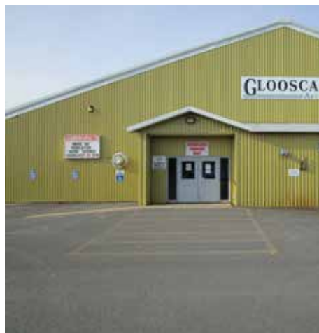
PA 4 | Accessible parking at Glooscap Arena
