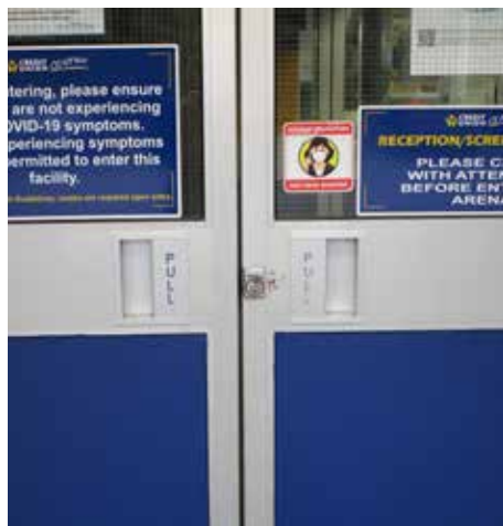
WS 1 | Credit Union Centre front entrance doors
