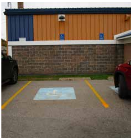
PA 2 | Credit Union Arena Accessible parking
