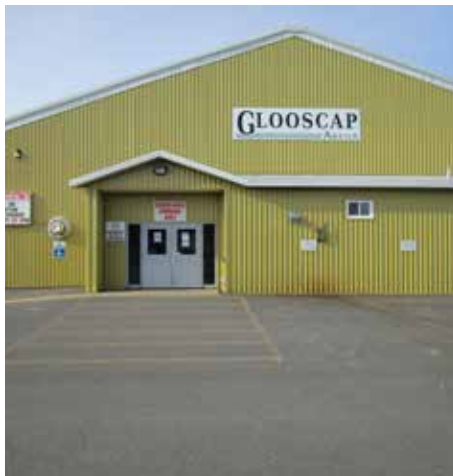
KA 4 | Front entrance to arena
