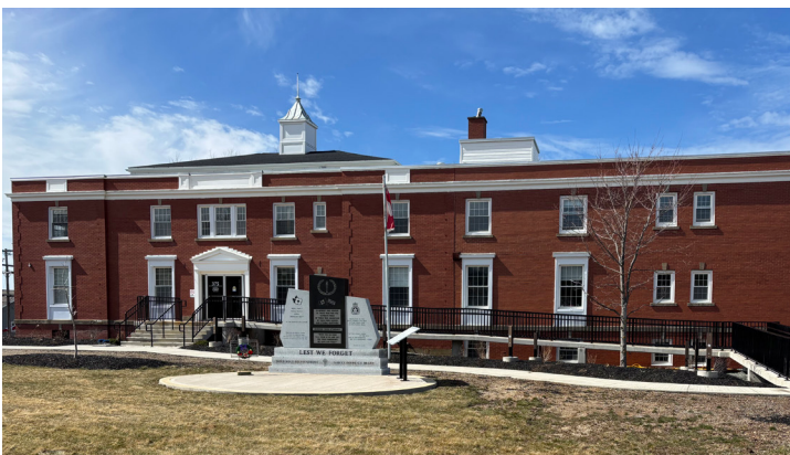
Photo: New accessible entryway at the Municipal Administration Building, Port Hood
